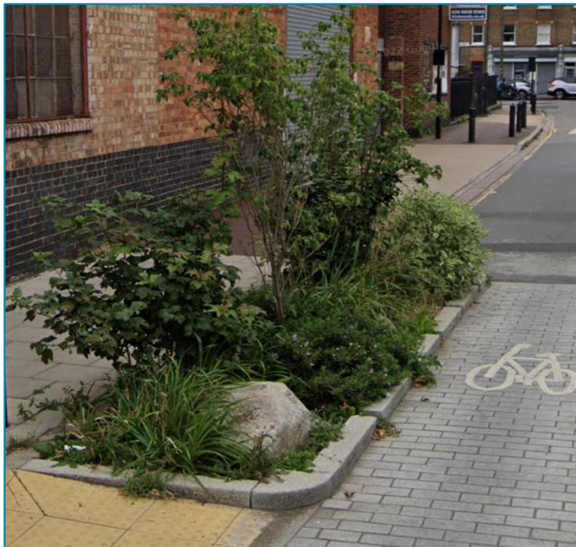
Figure 5-32: Sample Rain Garden Kerbing Inlet Layout
