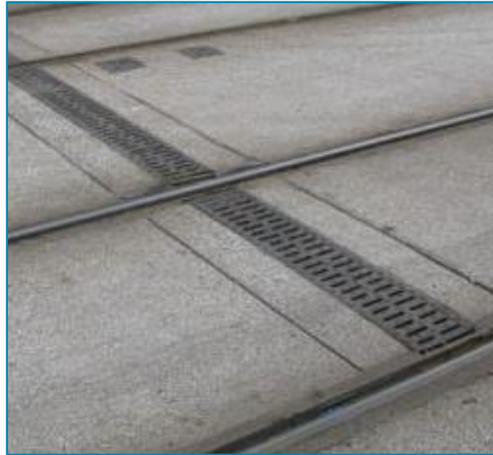
Figure 5-30: Detail of Slot Drain Collection Channel
