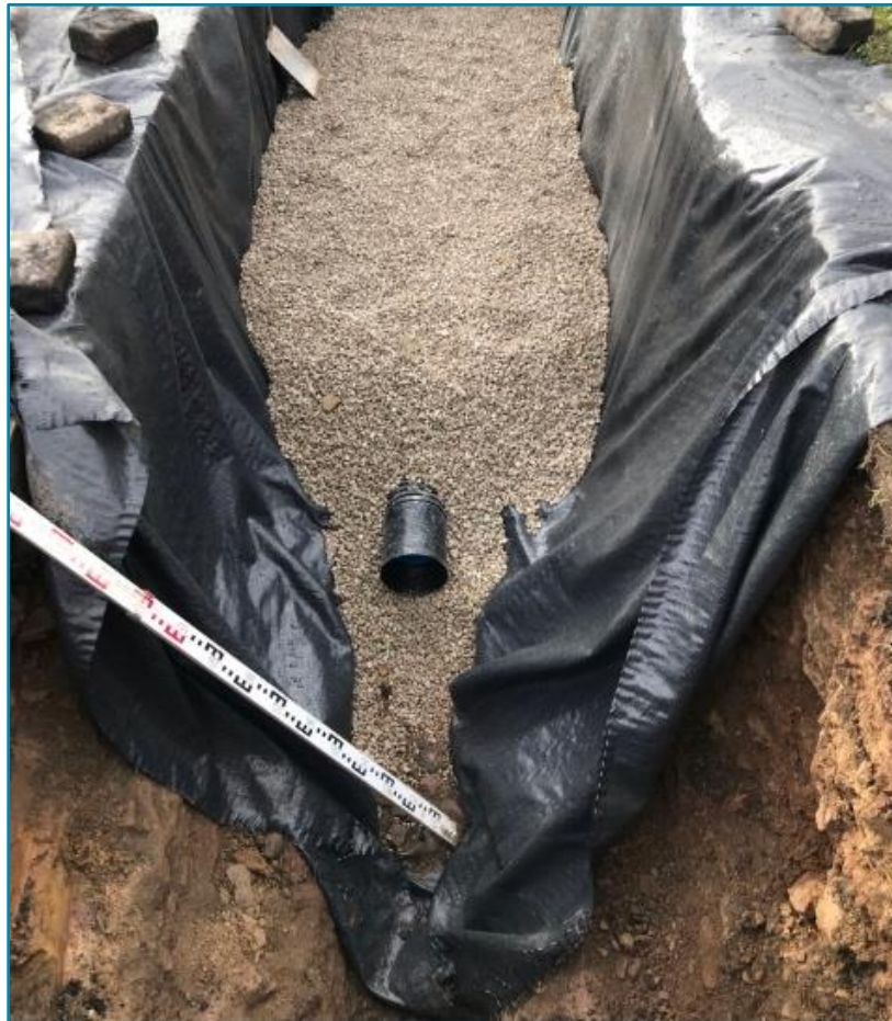
Figure 5-33: Rain Garden Construction
