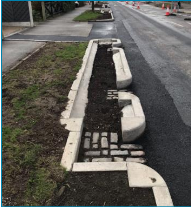
Figure 5-31: Sample Bio-retention Rain Garden Kerbing Inlet Layout
